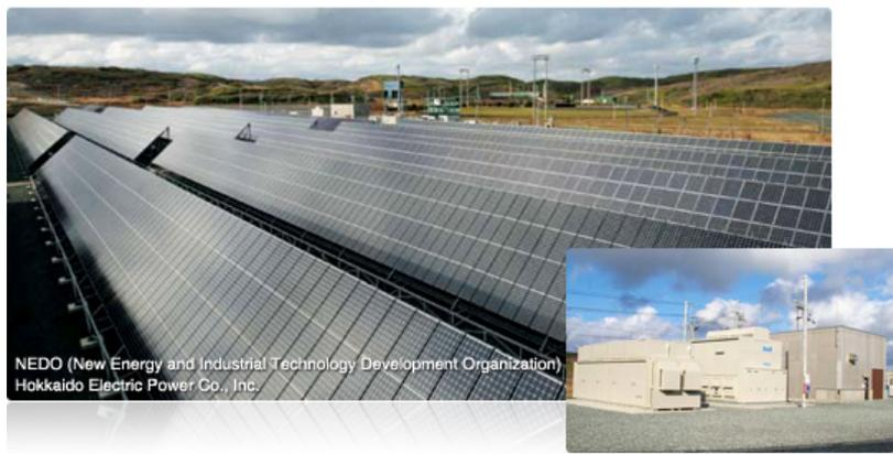
**Figura 5.5 1.5 MW NaS in 5 MW Solar PV Array**
