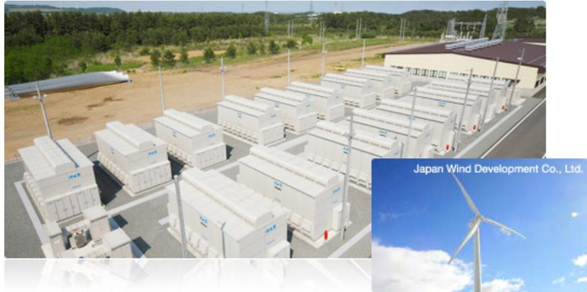
**Figura 5.4 34 MW NaS in Wind Farm da 51 MW**
